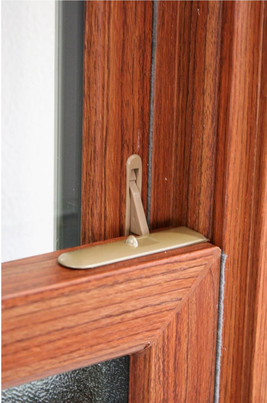
The Night Latches can be found at the bottom of both sides of the top sash of your Double Hung Window.
