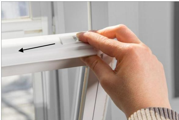
To tilt the sashes engage the Tilt Latches, which can be found on both sashes on the top at each side. Simultaneously slide both latches on the sash towards the center and you will be able to tilt the window.
